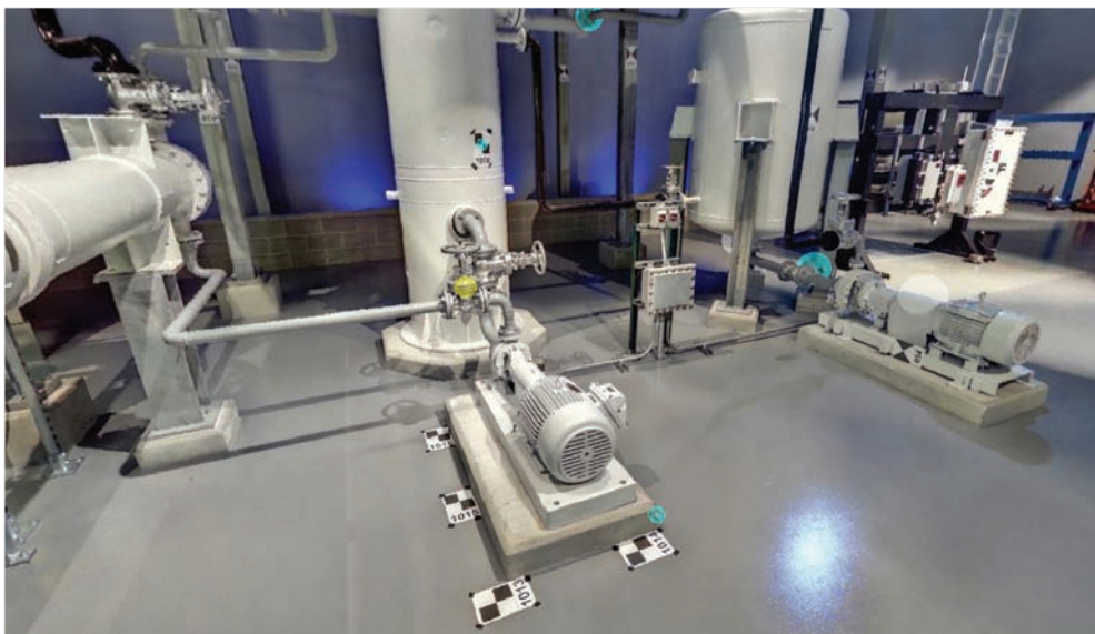
AVEVA LFM NetView provides a window into your point cloud data. The BubbleView gives you a scanners eye view in which 3D data can be measured and intelligence added to it.
